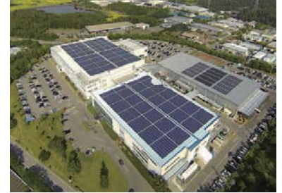
On-site use of solar energy (Photo shows Fujiyama Works)
