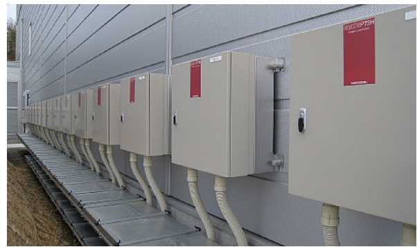
PV Inverters at Fujiyama Works
