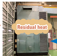
Indoor air handling unit (AHU)
