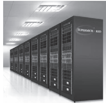
Fig. 1 Example of a rack mount server (Photo courtesy of Super Micro Computer, Inc.)
