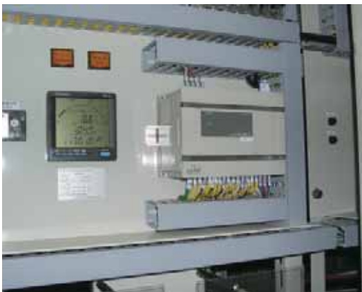
Energy measurement system
